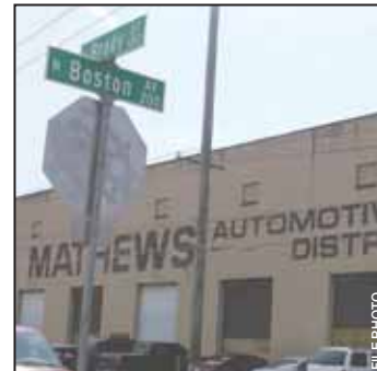
Sketch-Pad Dreaming. New plans for the Brady Arts District includes Brady Town Square and a geothermal well field to heat and air condition areas including Mathew Building.
